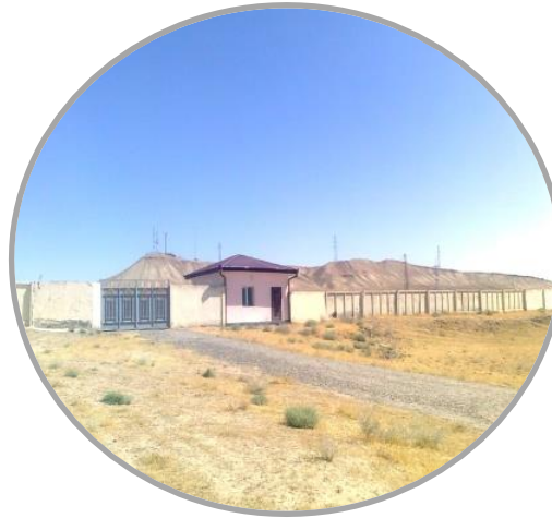
Water reservoir 1.0 thousand cubic meters.
